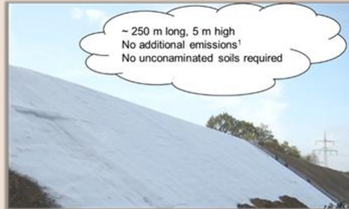
Sealed noise barrier wall
