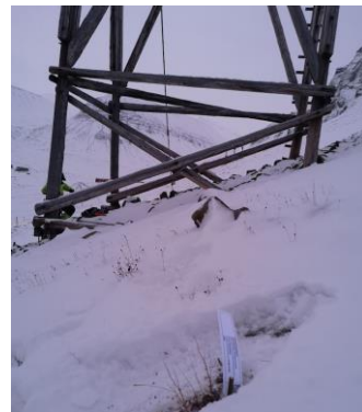
An i-button installed and marker with a shield. Picture: Enevoldsen, K.
