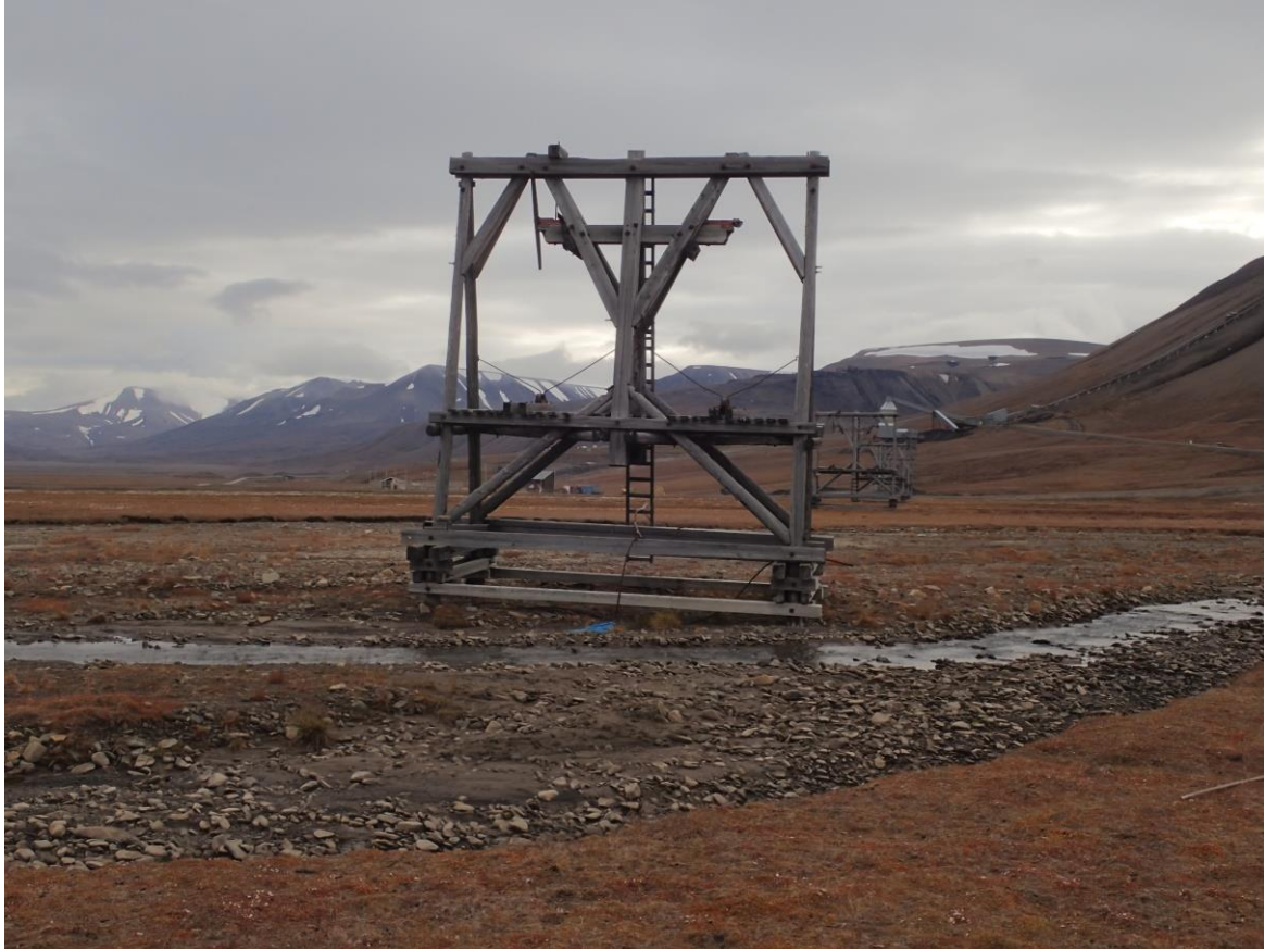
Line 6, Bukk 10 (pictures 10_1 and 10_2) – running water in seasonal creek warms up permafrost, tilt of structure towards a creek.
